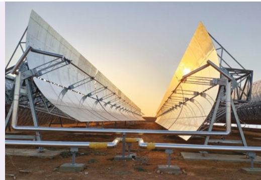
Mars Petcare Australia's Concentrated Solar Thermal system in Wodonga
