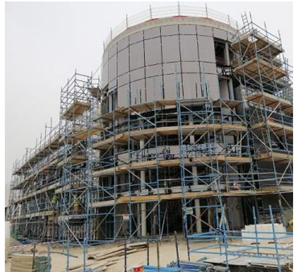
Expo 2020 Dubai: Fire Station
